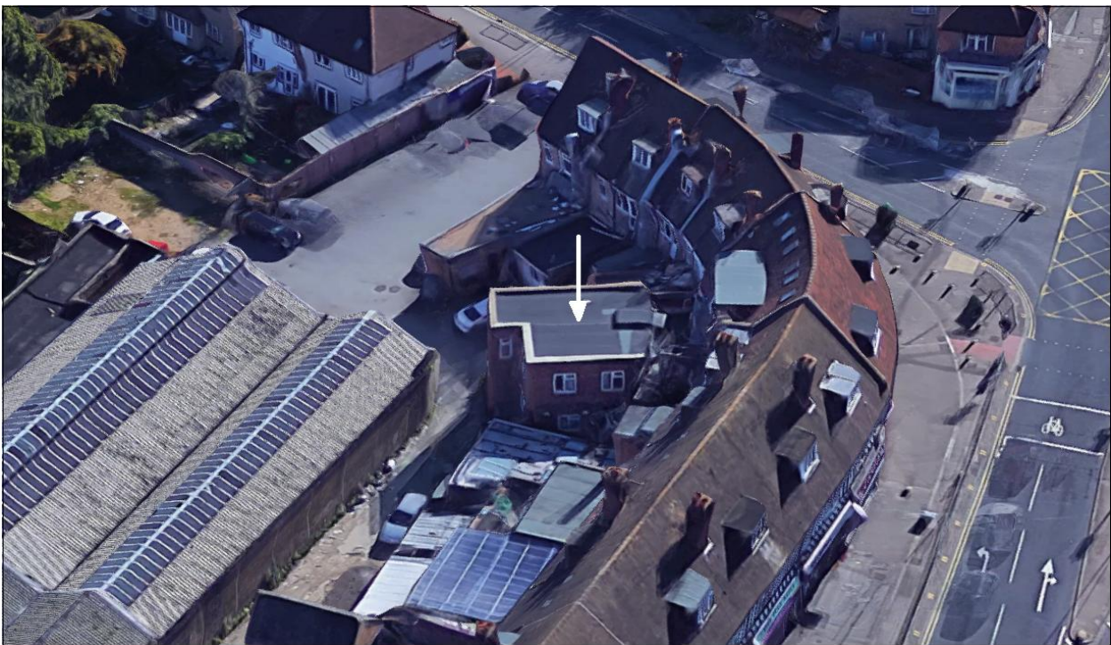
Fig. 1. Aerial view of site.
